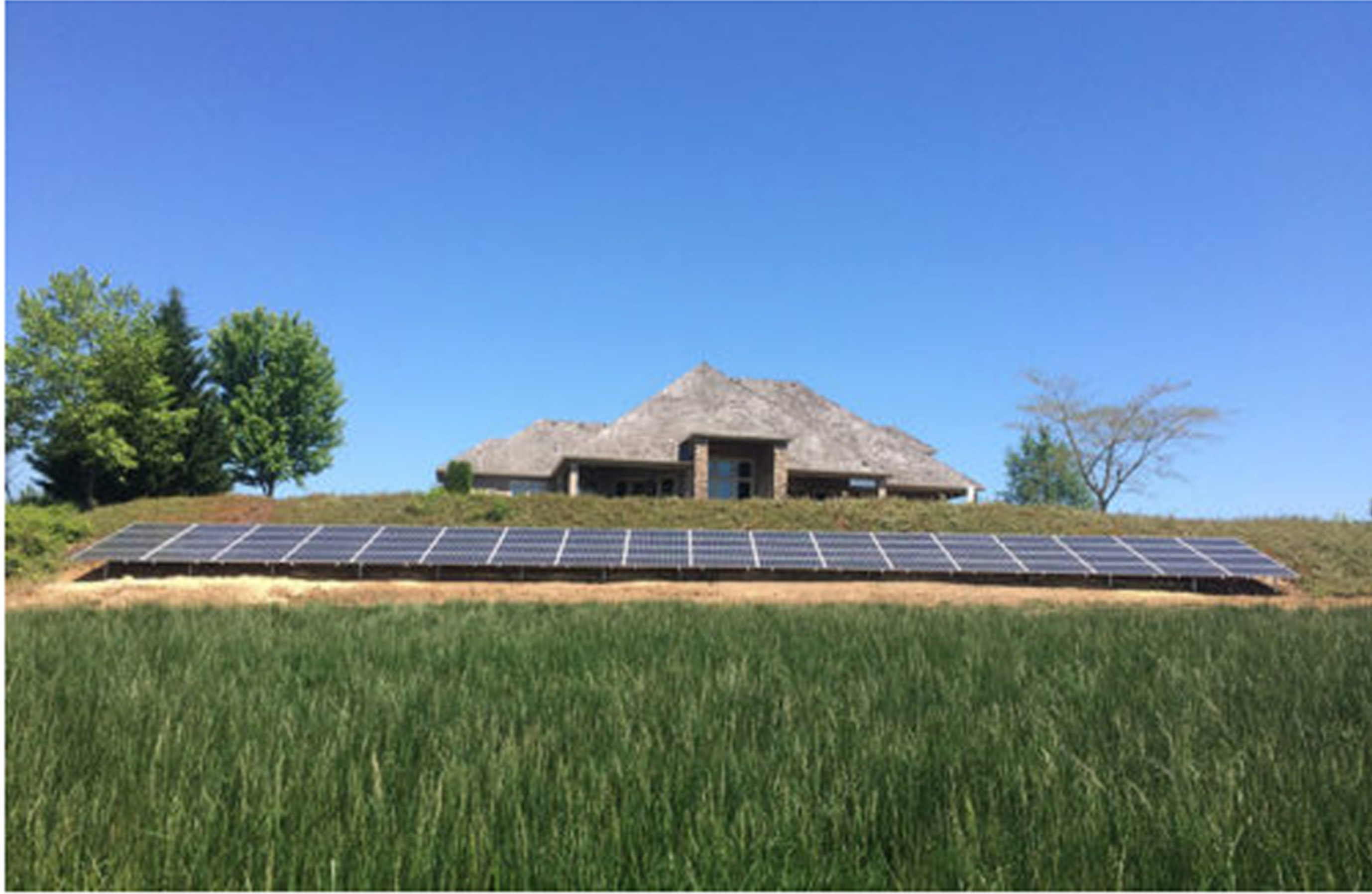
SunModo installed a residential ground-mount solar array into a hillside. SunModo.
