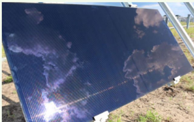
"Solar project in Florida, USA. Source: GameChange Solar ( www.gamechangesolar.com )"
