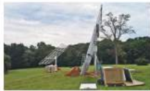
©2012 GameChange Racking, Inc. All rights reserved. Photo by GameChange Racking, Inc.
