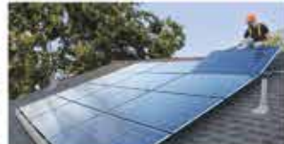
GC's Mounting Tray is used to set the system for correct mechanical loading and panel installation. It also features integrated grounding. Photo courtesy of GameChange Racking.
