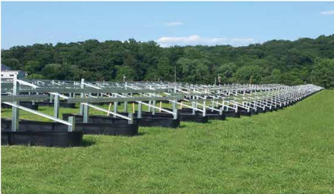
In the end, the result is a better rack at a lower cost. A rooftop system can come to 16 cents per watt (10 cents for materials, six cents for labor), far lower than the 25 to 32cents per watt outlined by GTM Research. Ground-based system for commercial and utility projects, meanwhile, can come in at 18 to 24 cents per watt, all-in.
